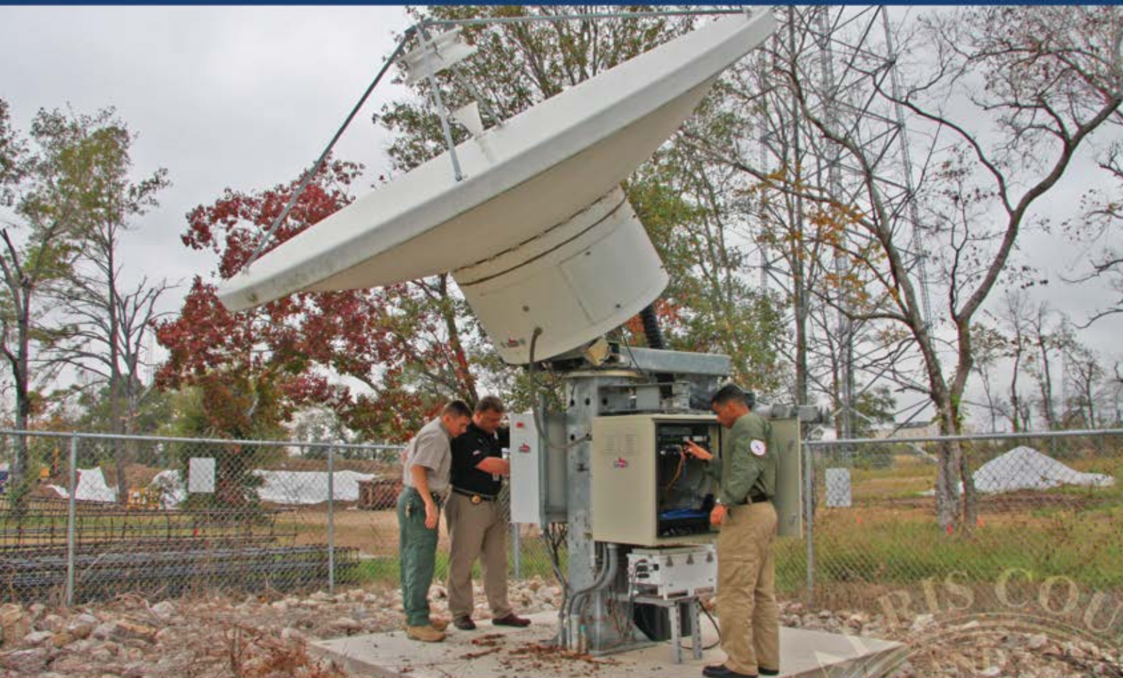
HCOHSEM logistics staff inspects satellite dish.
